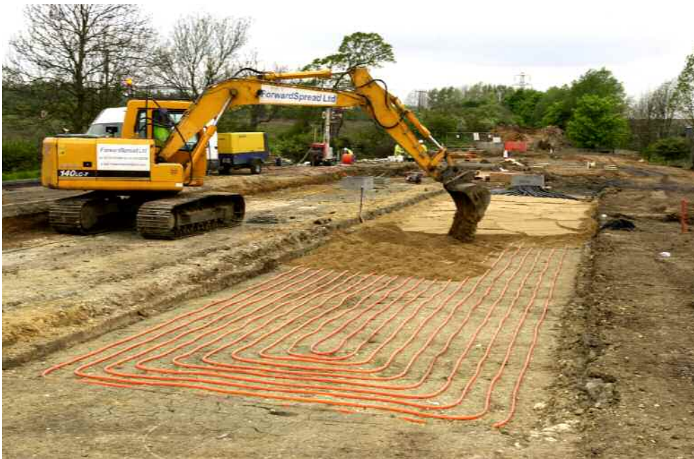
Figure 4.5. Placing sand over the off-road heat store
