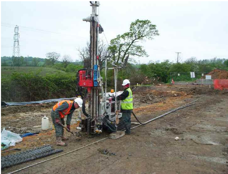
Figure 5.1. Rotary drilling for thermistor installations
