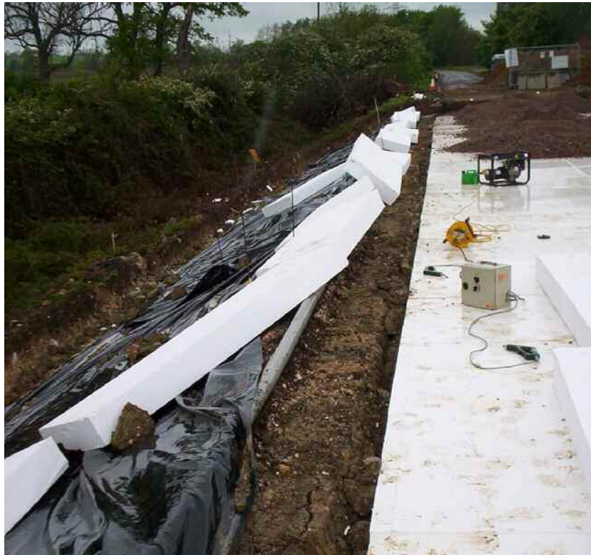
Figure 4.7. Polystyrene insulation being installed on the slope
