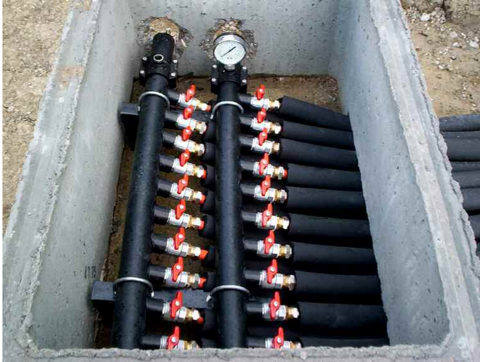
Figure 4.4. Manifold system within inspection chamber
