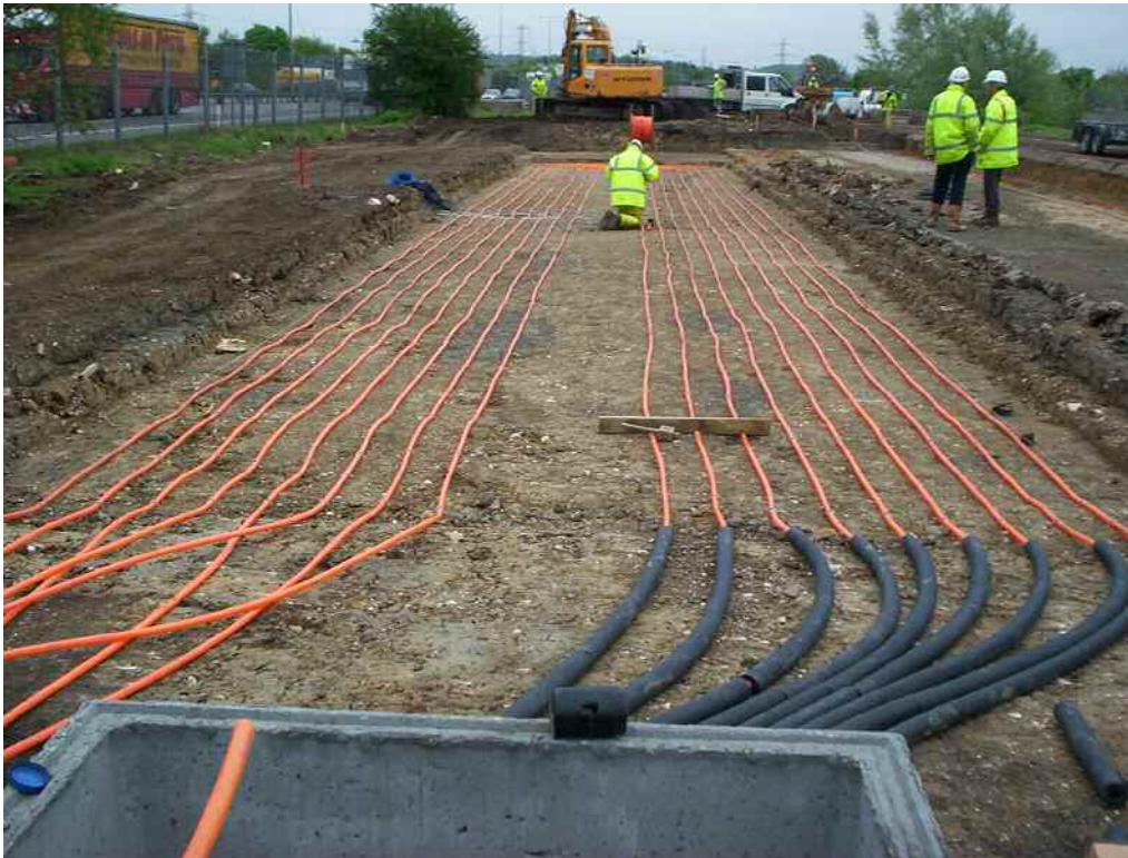
Figure 4.2. Pipework for off-road heat store being installed
