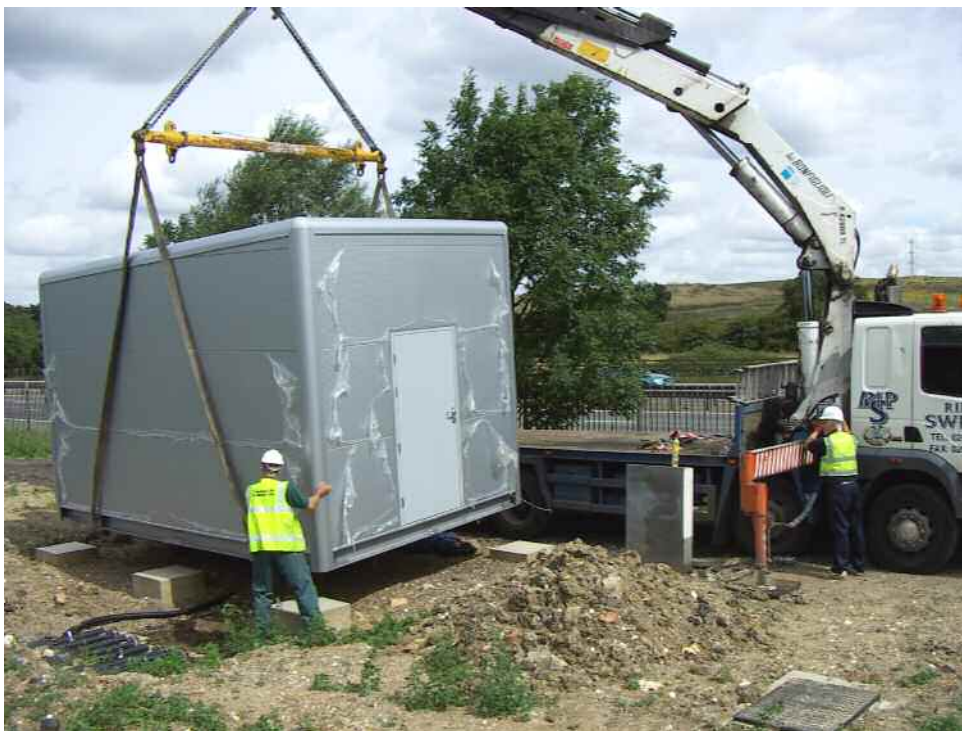
Figure 4.8. Pump house delivery
