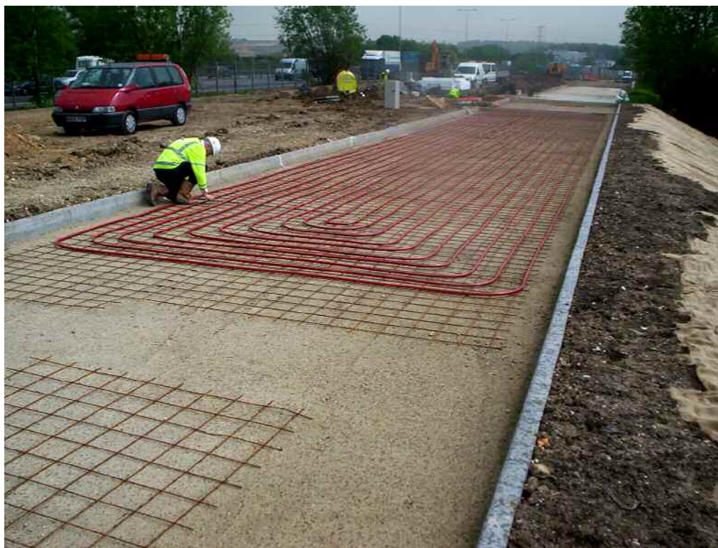
Figure 4.3. Completion of pipework for heat collector 2
