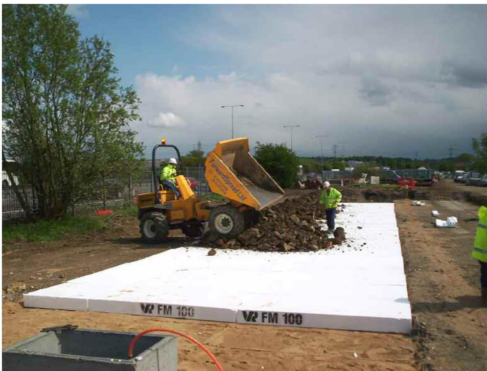
Figure 4.6. Placement of polystyrene over the off-road heat store
